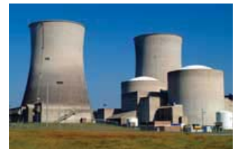
Watts Barr Nuclear Plant
